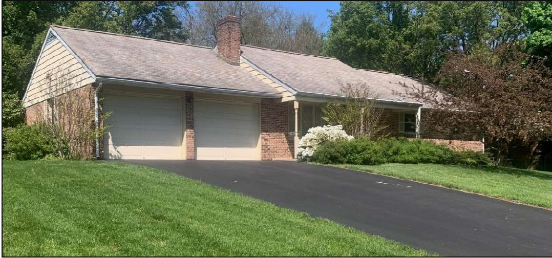
BRICK RANCH STYLE DWELLING WITH ATTACHED TWO CAR GARAGE (Approx. 1,320 sq. ft. Living Space)
